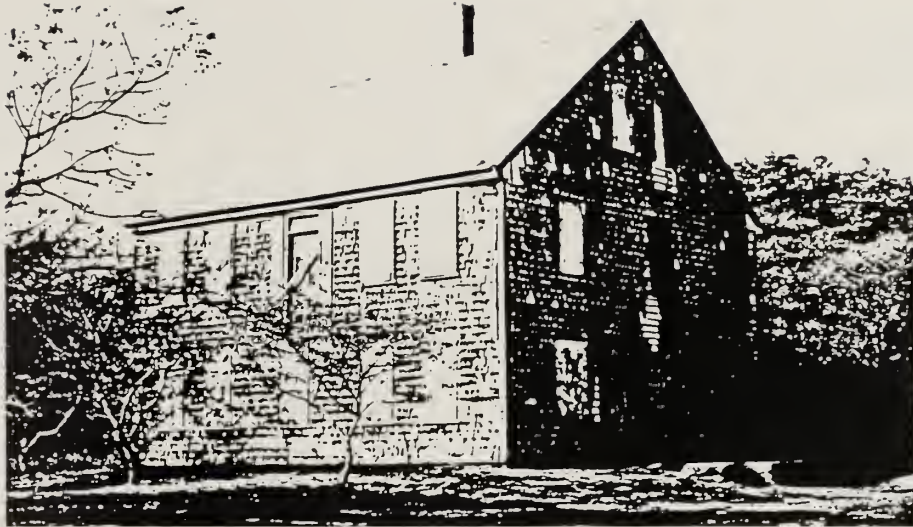
Bog House - Tract #17-2706 Bldg #T-17-23
